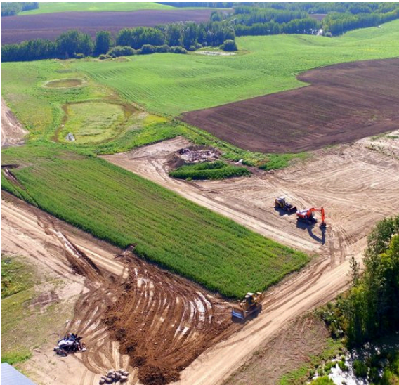
EARTHWORKS AT THE GROUP'S OWN TEST FACILITY, ALBERTA
