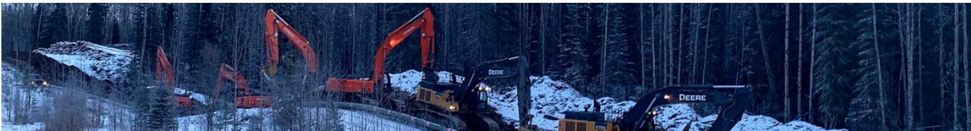
EXCAVATORS AT WORK ON A WINTER RIGHT-OF-WAY AT DUSK, WESTERN CANADA
